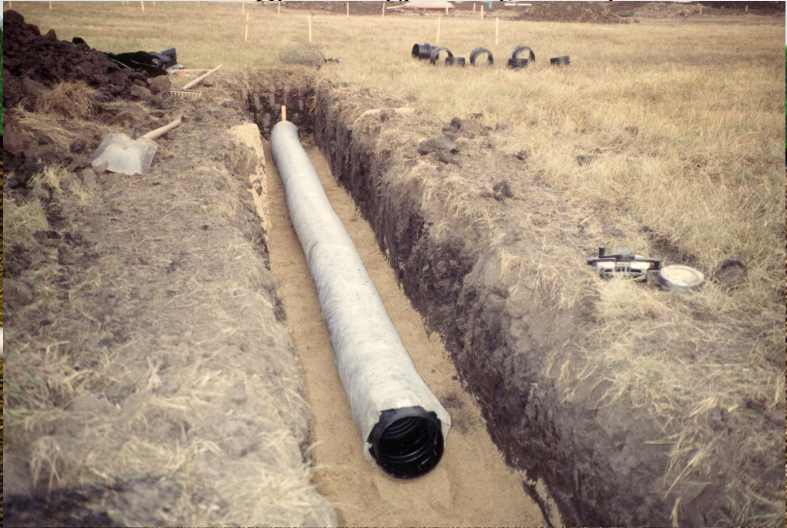
Soil absorption field
