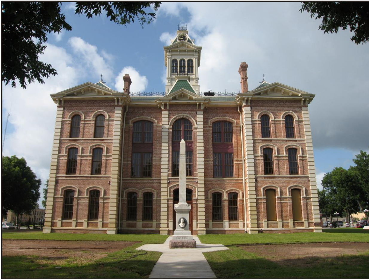
Wharton County Courthouse 1889 Wharton, Texas
